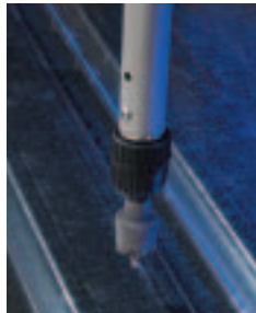
Drill Deck Holes
